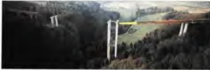
Fig. 1. Launching of the north bridge. February 1998. Photo courtesy of IABSE.
